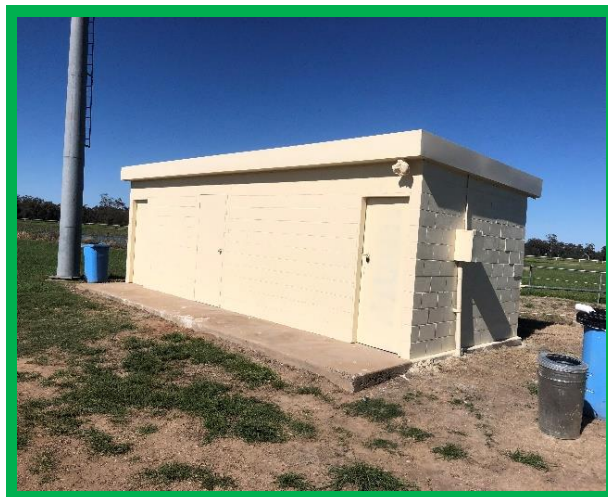
Centre Showground Arena Toilet Block
