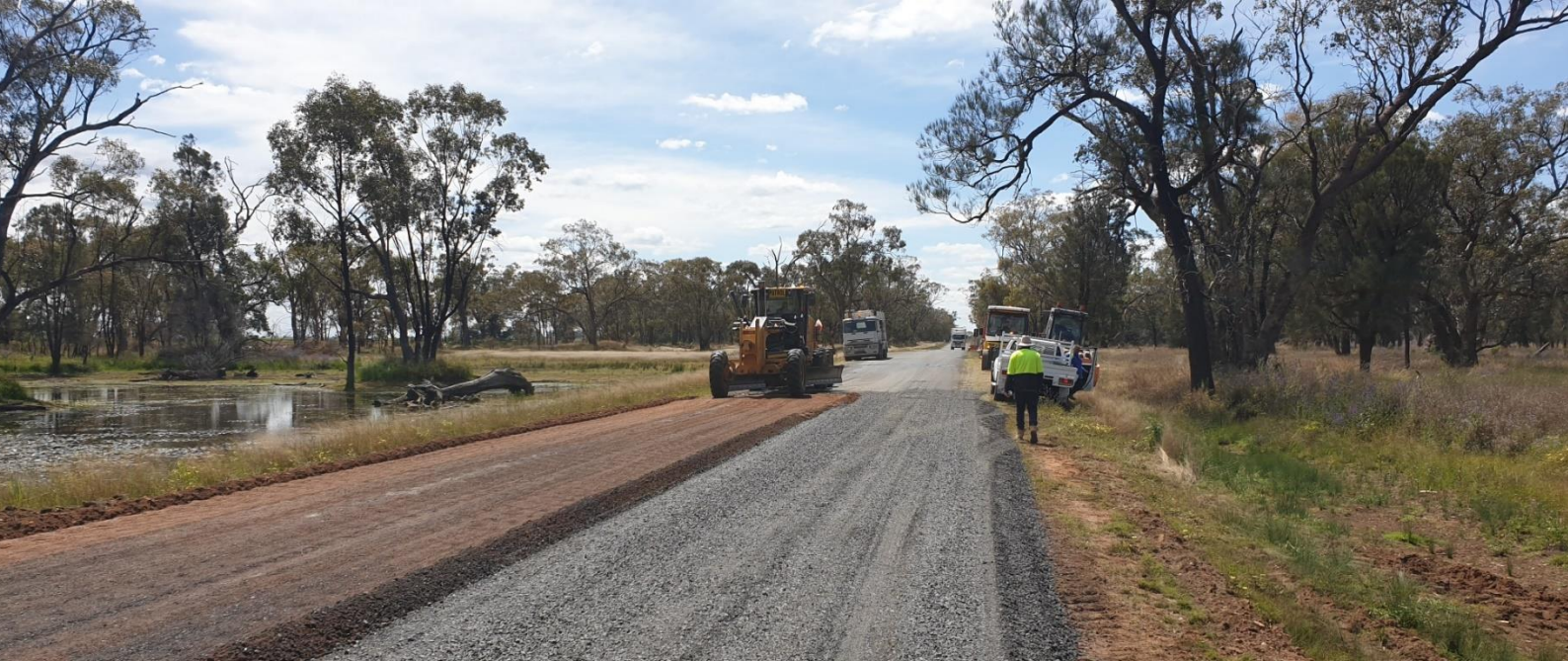
Heavy Patching RR 7515 –Warren Road
