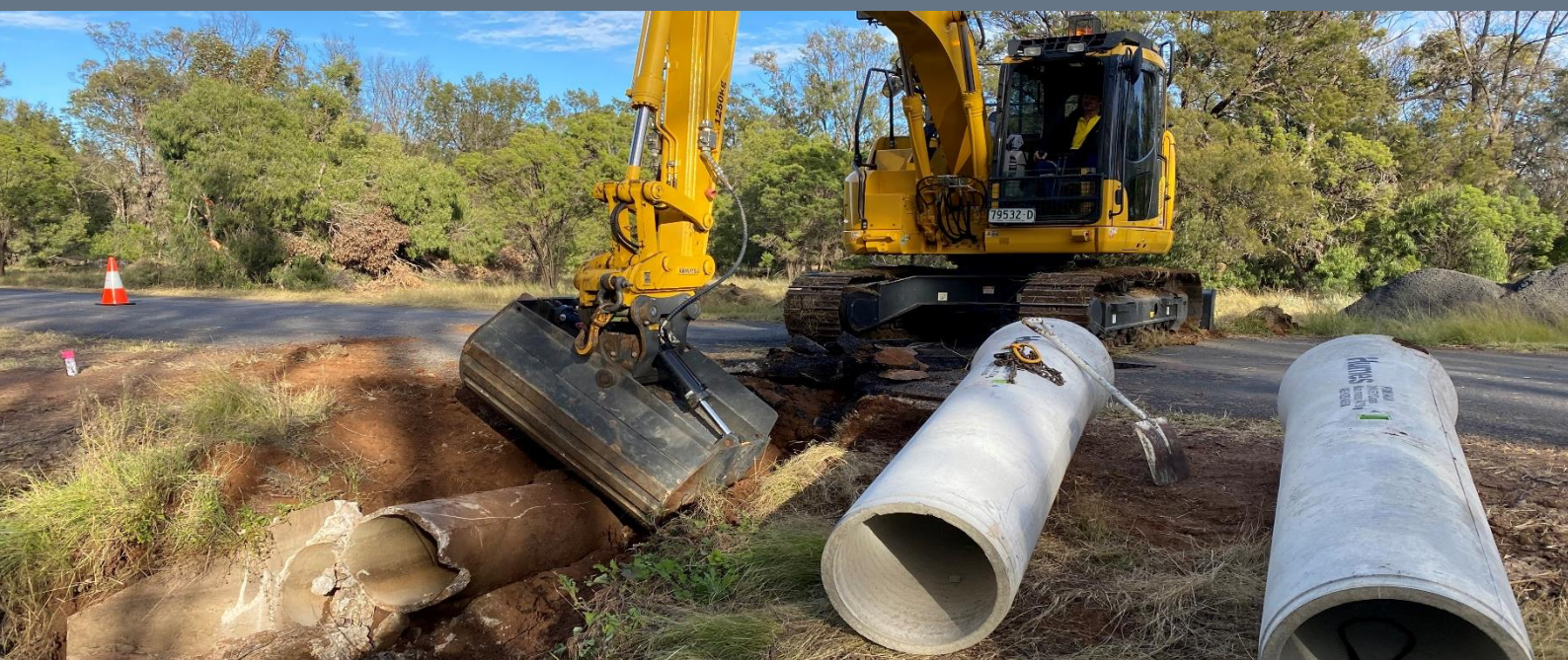
Replacing Culverts Collie – Trangie Road
